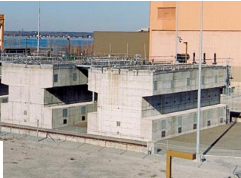
After several years in water bays and when the radioactivity has diminished considerably, nuclear fuel can be stored in concrete containers like these. This material is stored for eventual permanent disposal.
