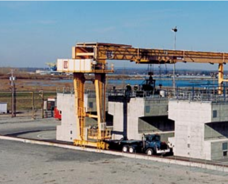
After several years in water bays and when the radioactivity has diminished considerably, nuclear fuel can be stored in concrete containers like these. This material is stored for eventual permanent disposal.
