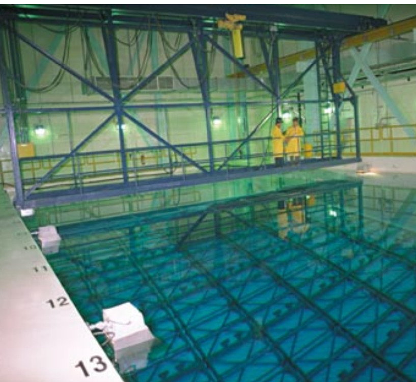
Used nuclear fuel is stored in water bays within each of Canada's nuclear power stations. Here the used fuel can be monitored and cooled.
